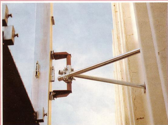
Easily fixed mast ties.
